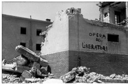
Inscription on the wall of a bombed building, translated as “Work of the Liberators”
